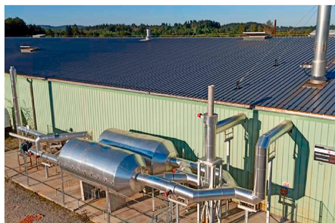
Fig. 5. Industrial installation of the Eco-Stock® thermal storage system.
